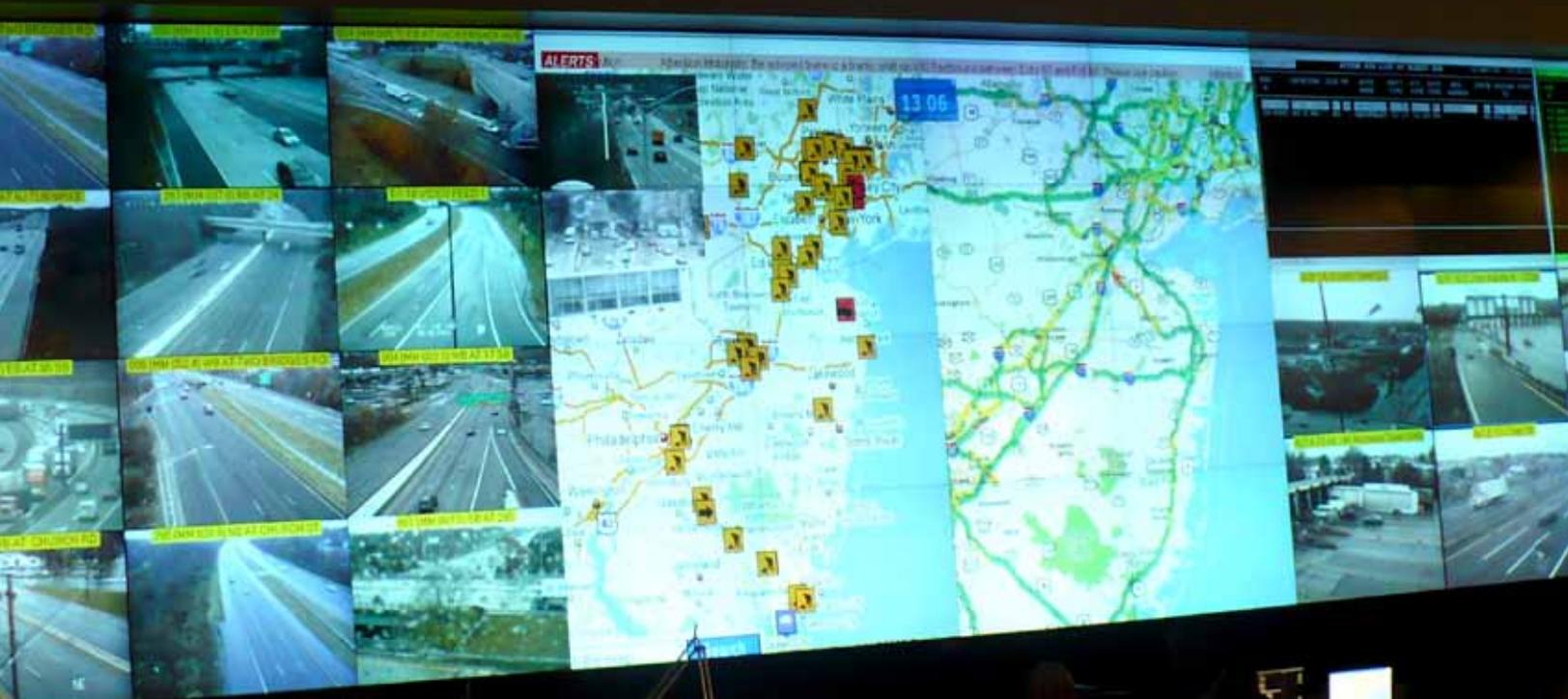
The New Jersey DOT Command Center uses INRIX real-time data and analytics to monitor congestion and deploy resources proactively to manage traffic flow and inform travelers.
